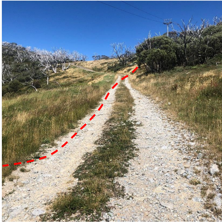
Photo 3: Part of the trench will be through the previously disturbed Norwegian Road, which will be reinstated to a trafficable access track.
